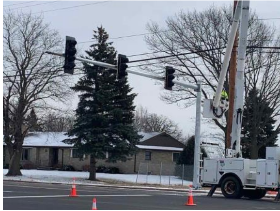
New traffic lights are installed in County Hwy II (12/07/2021)
