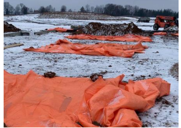
Special blankets are used to insulate the ground to help prevent frost where concrete footings will go (12/09/2021)
