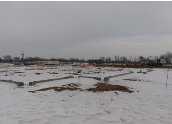
Completed concrete foundations in the Northmost classroom wings (12/29/2021)
