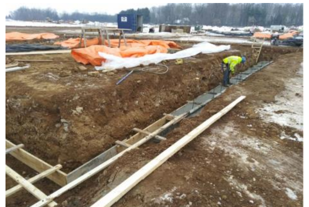
Concrete footing forms are prepped prior to being poured (12/29/2021)
